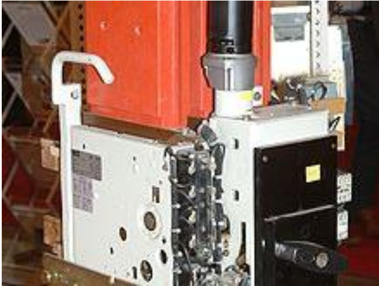
An air circuit breaker for low voltage (less than 1000 volts) power distribution switchgear
